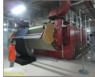
Photo of the inside of the main production hall Dyeing finishing section.JPG
