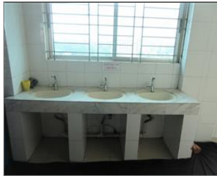
Photo of the inside of the main production hall Hand wash facility in dining area.JPG
